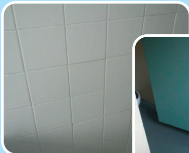
Grout re-whitened as standard
